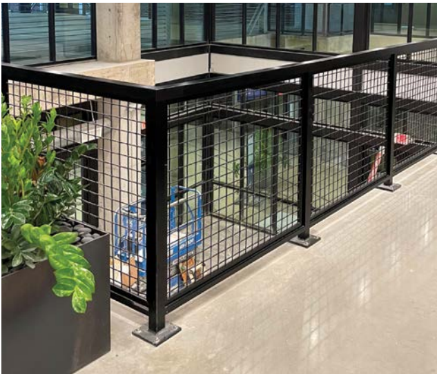
WIRE MESH PANEL INFILL RAILING
